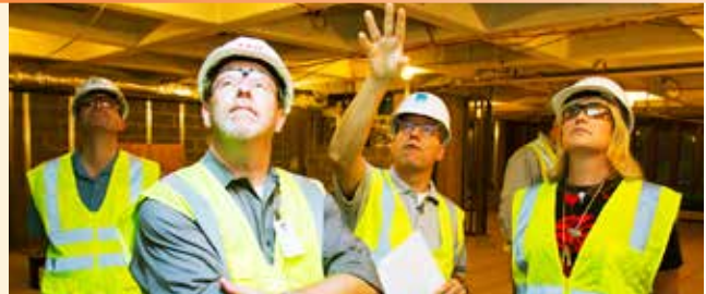
Deputy Managing Director Carla Grasso (right) inspects progress on HQ1 renovation.
